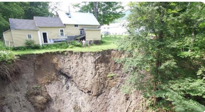
Flood Hazard Mitigation Project, Rockingham Landslide
