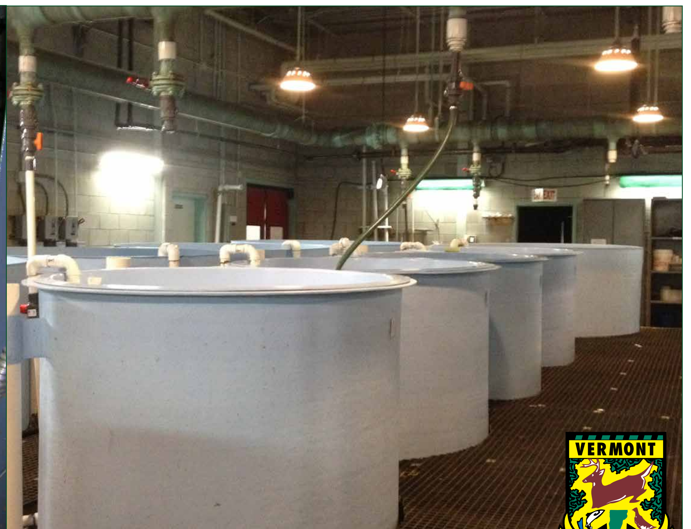
Recirculating previously heated water drastically reduces the amount of propane needed at Ed Weed hatchery to heat water for raising fish during the winter.
