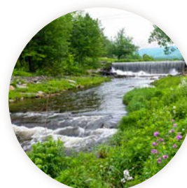
Water, Sewer, and Wastewater Infrastructure
