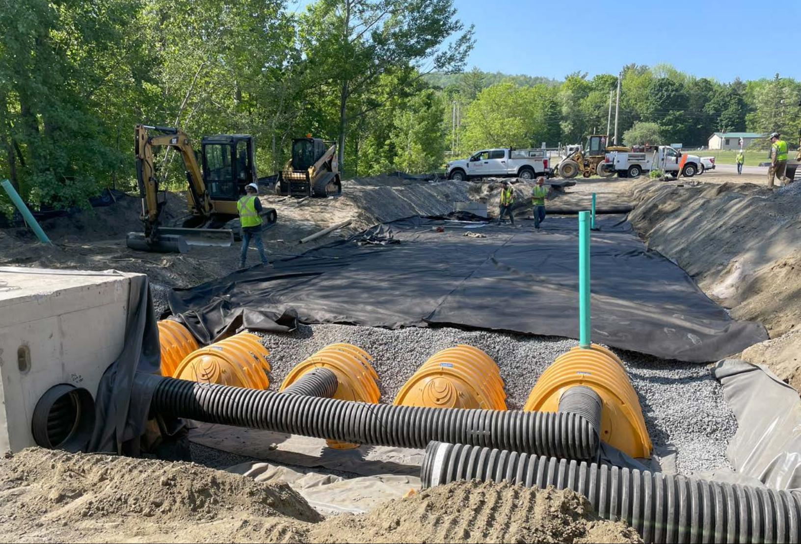
Barre Town Stormwater Mitigation Project
